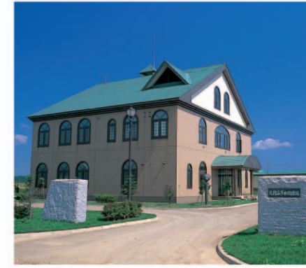
下水処理場〈北檜山区〉 Sewage treatment facility (Kitahiyama district)
