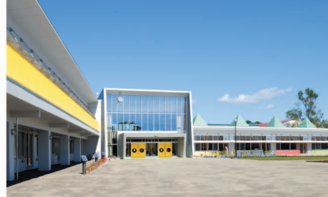
北檜山小学校(北檜山区) Kitahiyama Elementary School (Kitahiyama district)
